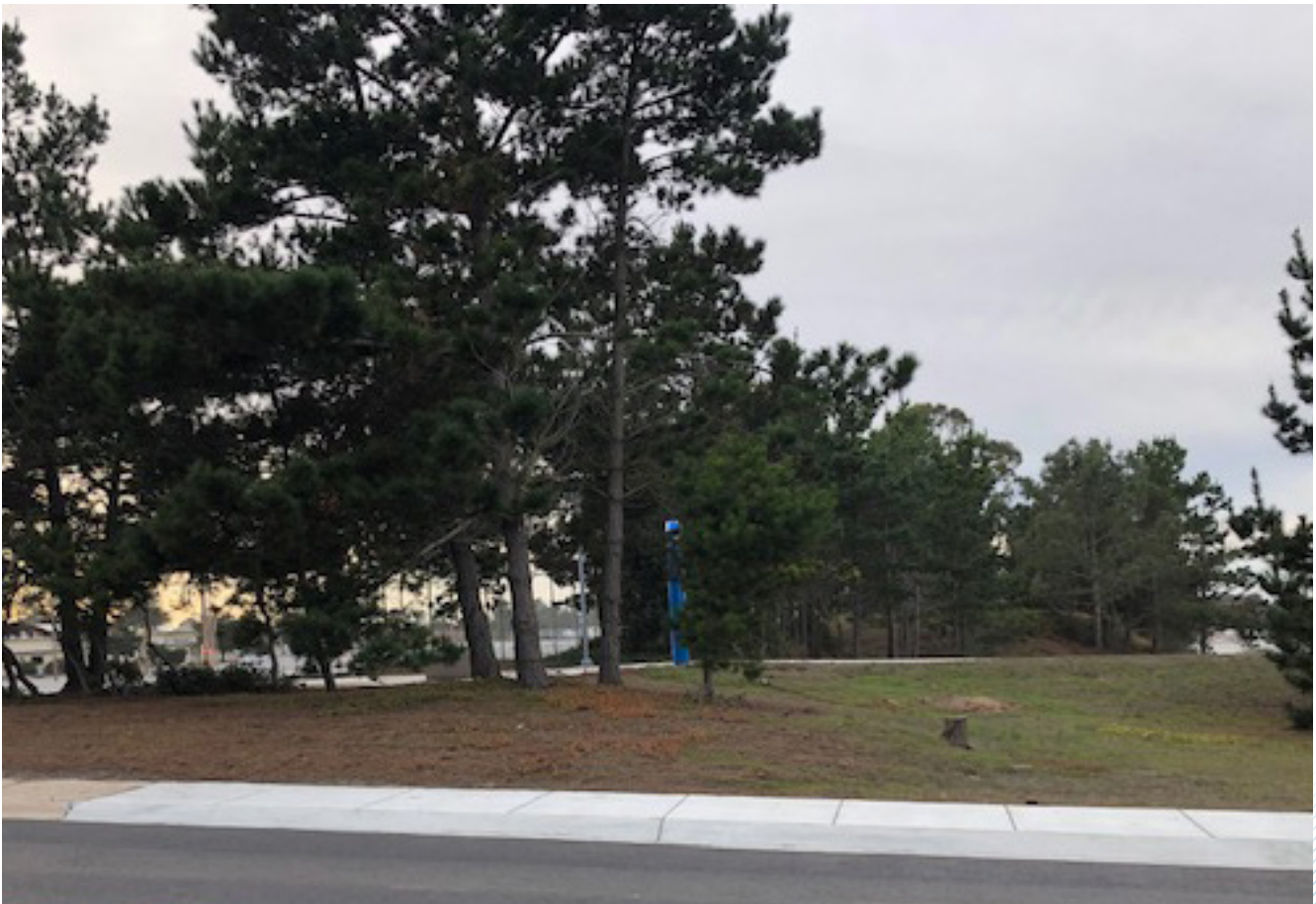
A Zone and C Zone Pipeline Alignment from 6th Ave. to Booster Pump Station Site.
