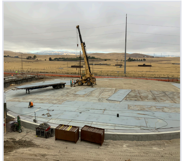
5 MG Tank - Tack Welding Floor and Annular Ring
