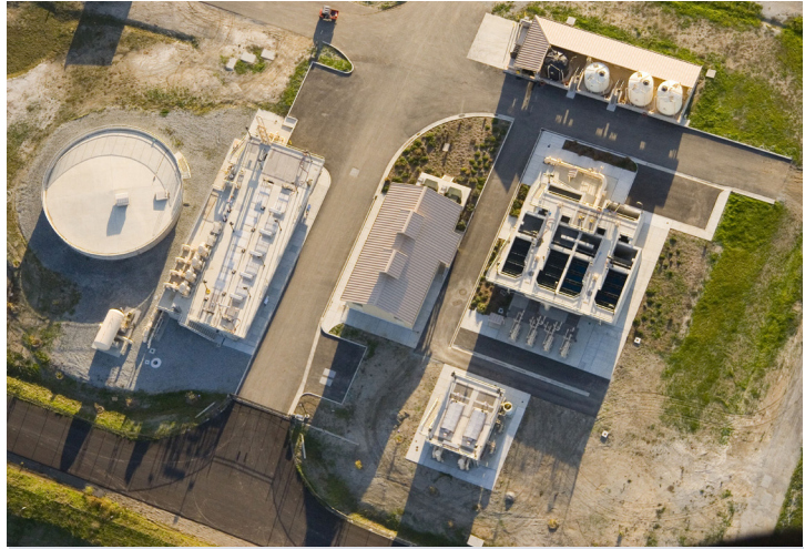
City of Watsonville Recycled Water Facility
