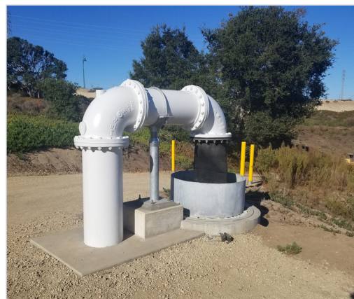
Percolation Basin Outfall
