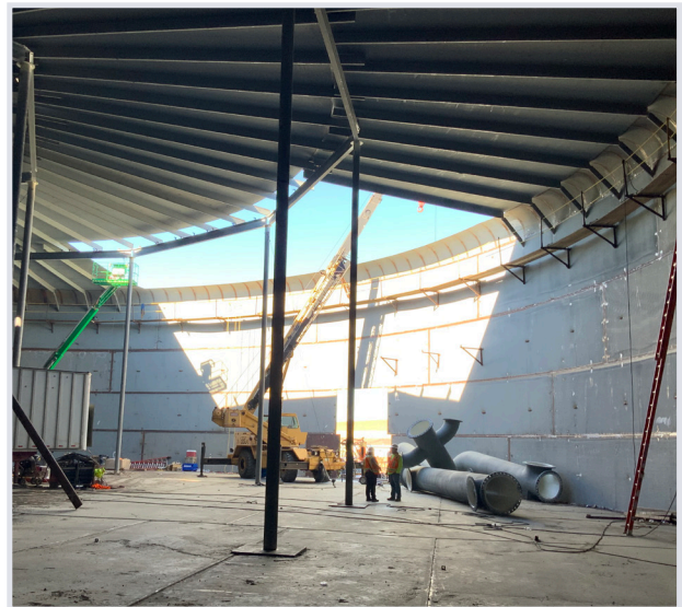
5 MG Tank - Building the Clearwell
