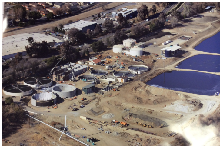
City of Paso Robles Wastewater Treatment Plant Upgrade
