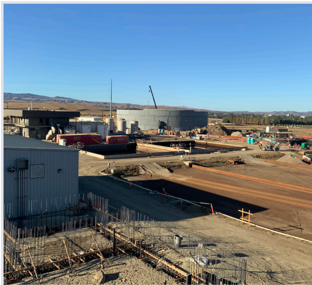
5 MG Tank - Welding on Top Radius of Clearwell
