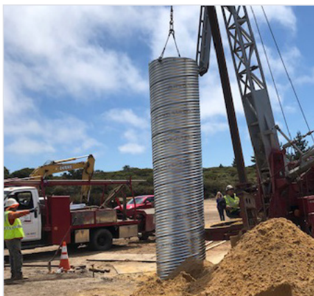
Injection Wells-2 Project - Well Construction
