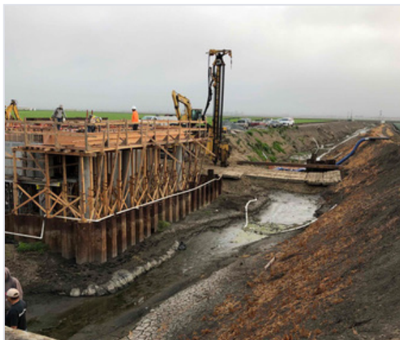
Blanco Drain Pump Station
