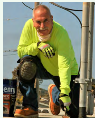
Regular maintenance at Well 10.
