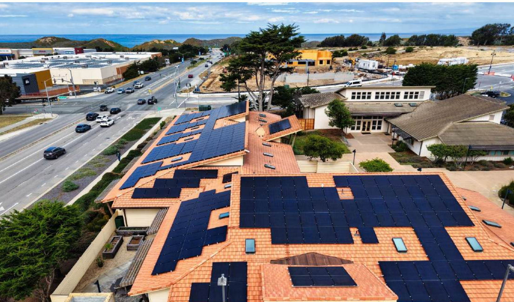
Top/Right: Aerial view of the Imjin Office Park solar array—expanding renewable energy capacity and supporting energy independence. Bottom/Left: Solar and battery storage system in operation—enhancing resiliency and providing reliable backup power for critical District facilities.
