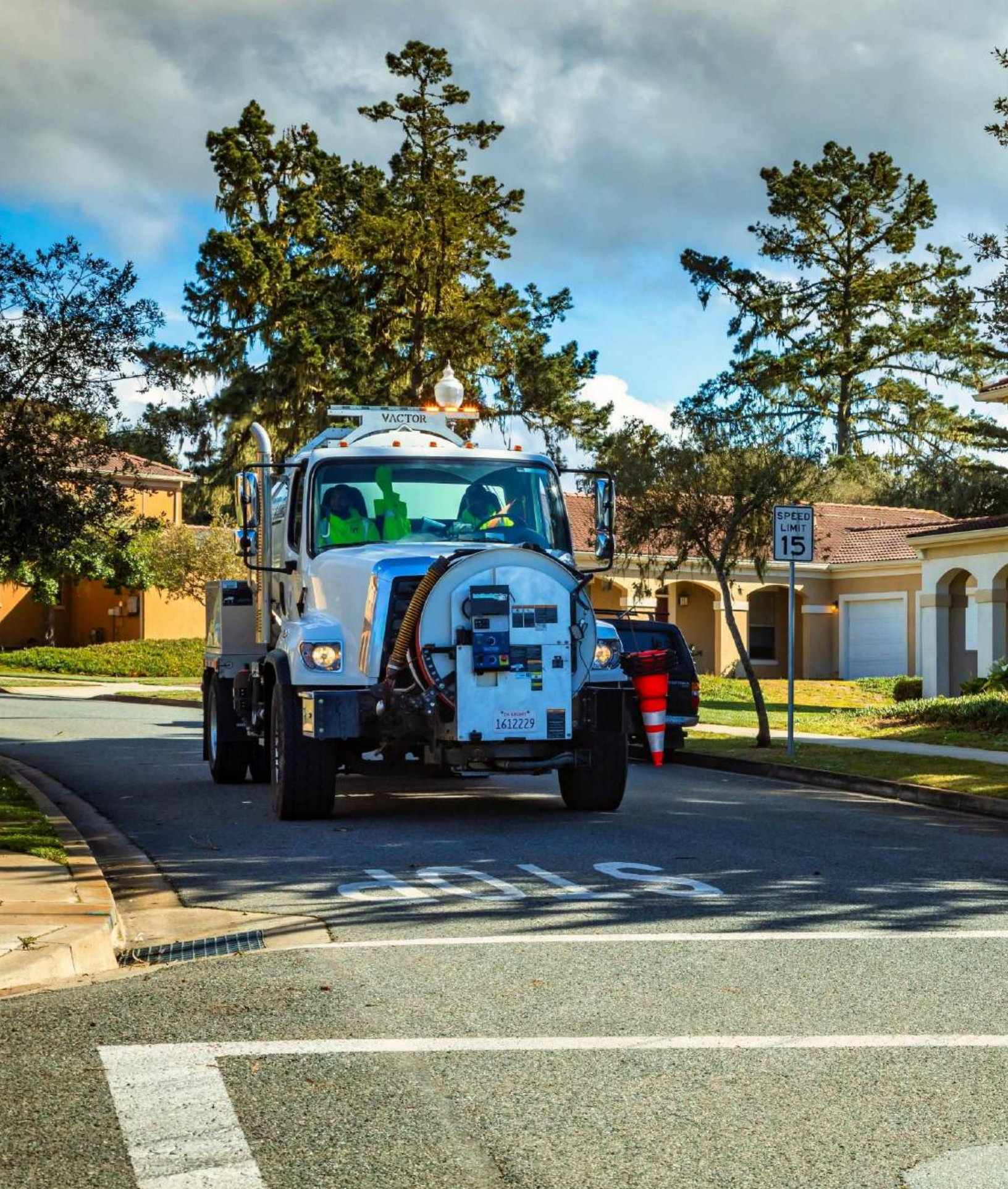
Field crew in action—maintaining and cleaning the system to keep service safe, reliable, and flowing smoothly.
