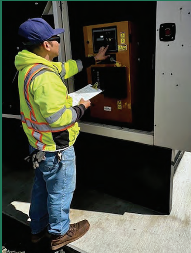
(Left) Operator exercising generator to ensure uninterrupted service during a power outage. (Above) Operator testing backflow device to ensure proper function.
