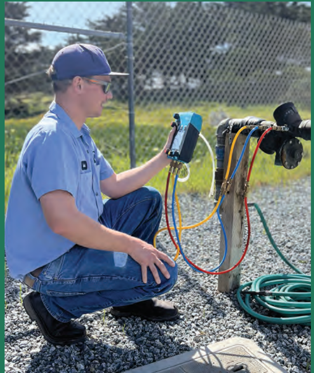
(Left) Operator exercising generator to ensure uninterrupted service during a power outage. (Above) Operator testing backflow device to ensure proper function.
