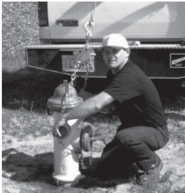
MCWD Distribution Operator Richard Green replaces fire hydrant.
