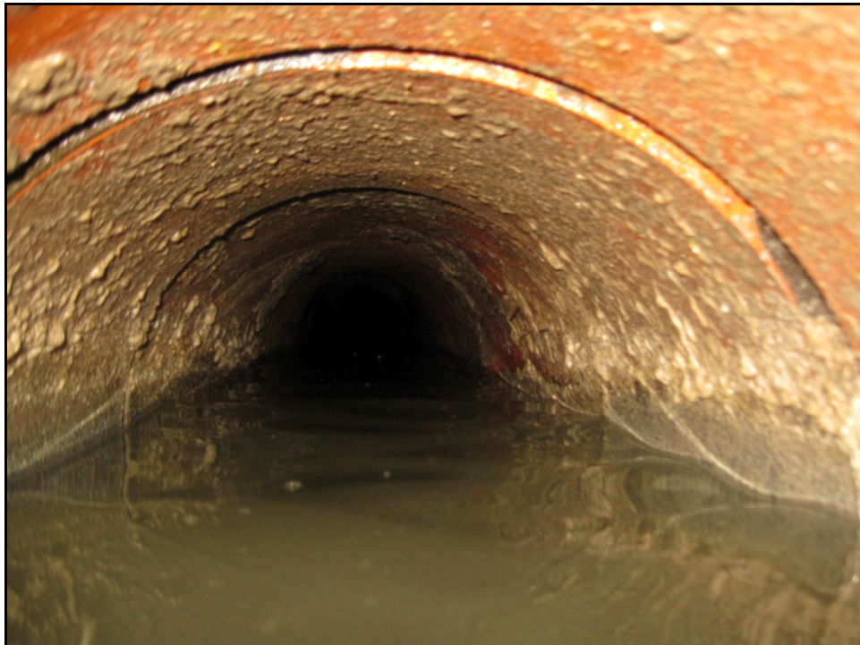
East Influent Pipe
