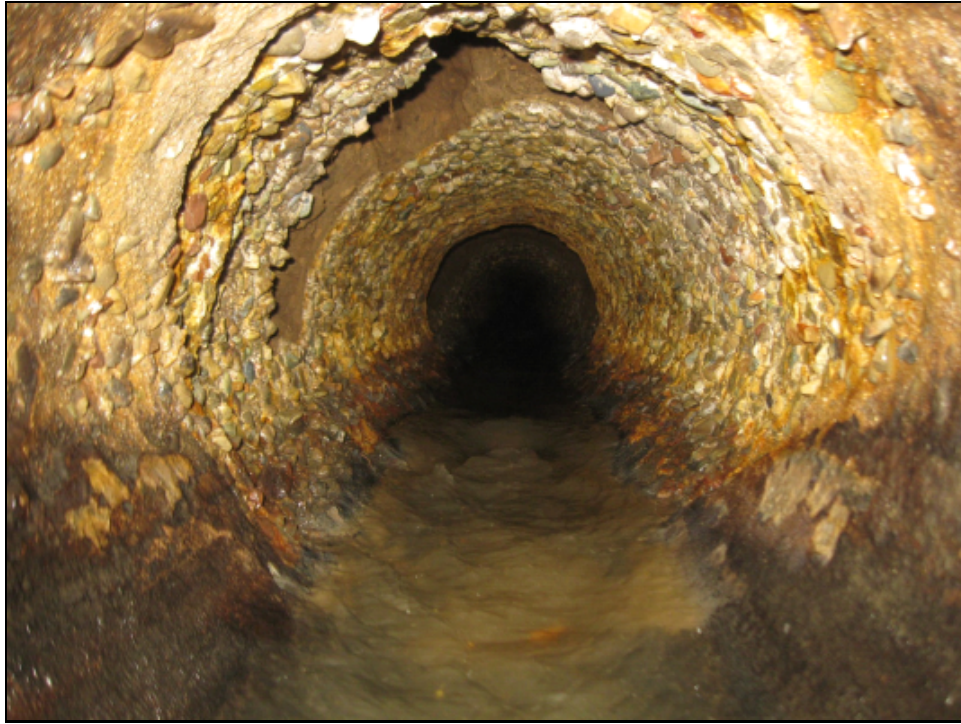
East Influent Pipe
