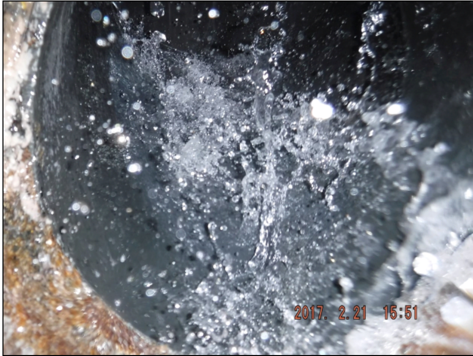
East Influent Pipe (Lower)
