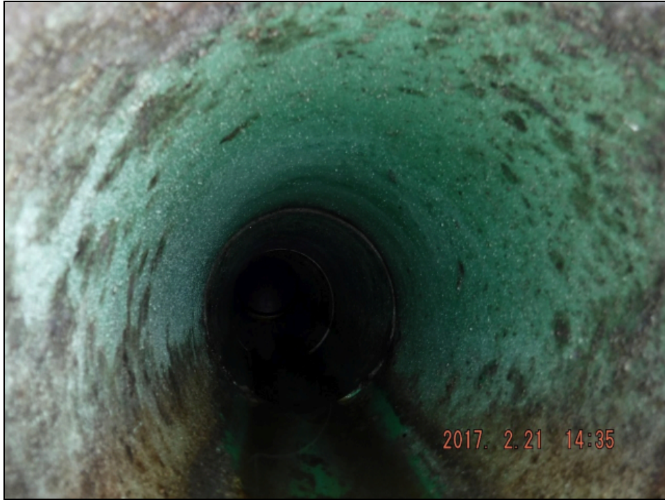
East Influent Pipe
